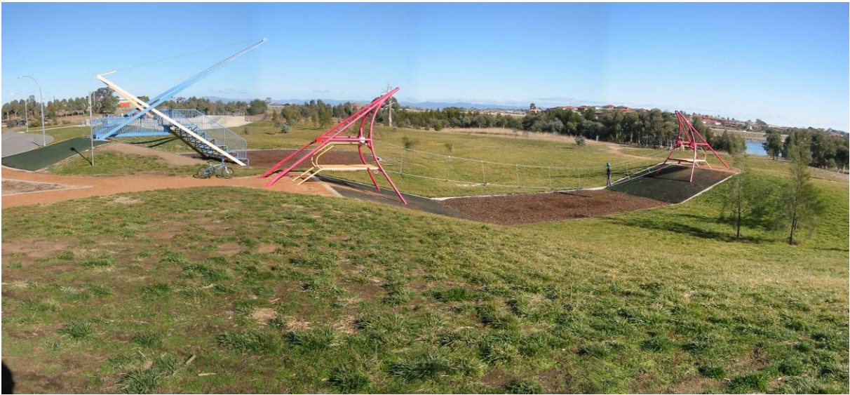
View of Yerrabi Pond District Park looking south west
