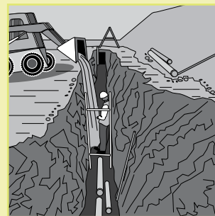
Figure 24: Example of an unguarded trench.
