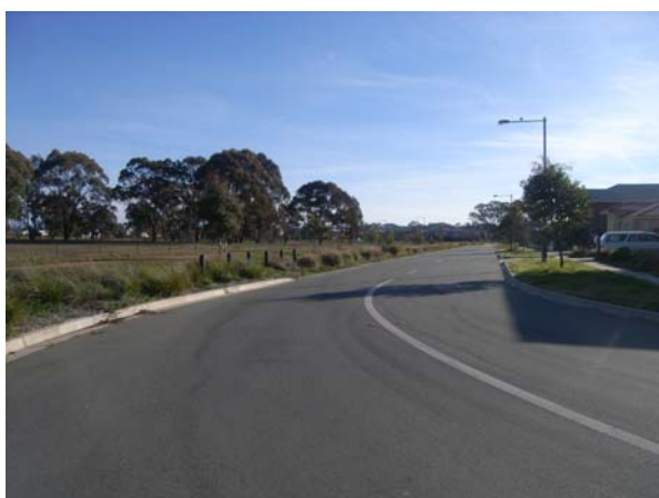
Figure 11.1 A sealed edge road, Forde
