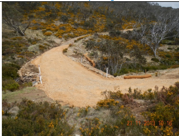
Stockyard Creek crossing on the upgraded section of Mt Franklin Road
