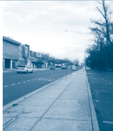
View southwards down Mort Street
