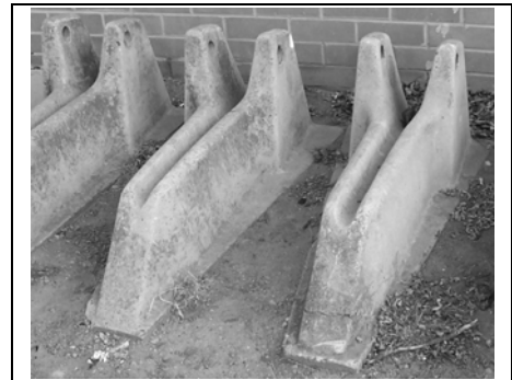
Figure 3 – An Example of Unacceptable Parking Installations
