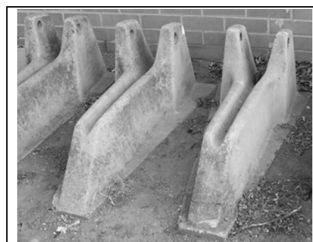
Figure 3 – An Example of Unacceptable Parking Installations
