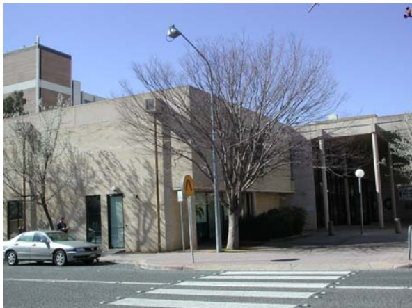
Figure 2. View from SW toward entry (EMA 2004)
