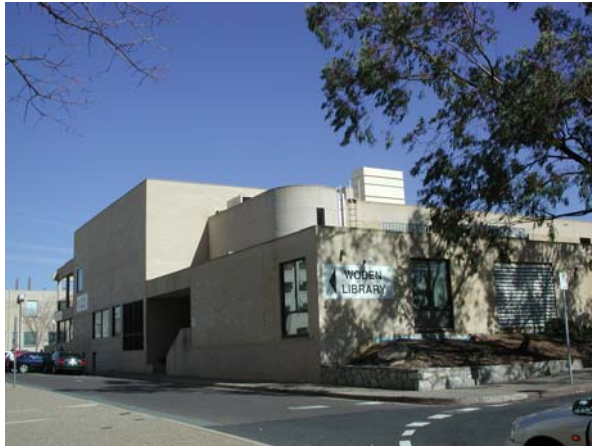
Figure 6. View from SW toward Entry (EMA 2004)
