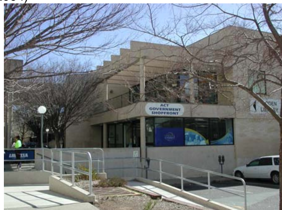
Figure 5. View from SW toward Entry (EMA 2004)
