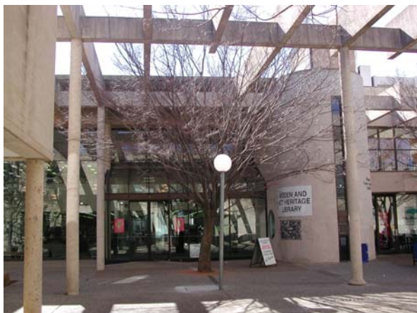
Figure 4. View toward Entry (EMA 2004)
