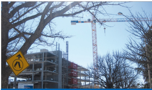
NEW COMMERCIAL DEVELOPMENT AT BARTON
