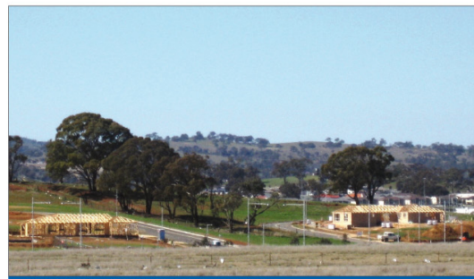
HOUSE CONSTRUCTION AT FRANKLIN
