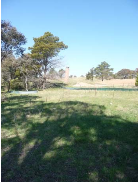
Ventilation Shaft (feature # 4)
