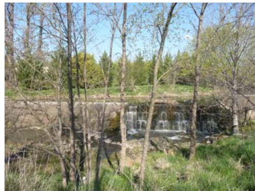
tunnel at Yarralumla Creek (sewerage tunnel forms part of the weir)
