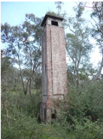
Ventilation shaft (feature # 36)
