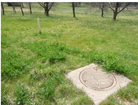
Access Chamber (feature # 37) in Stirling Park.
