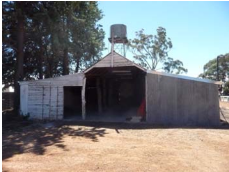
Machinery shed and water tank
