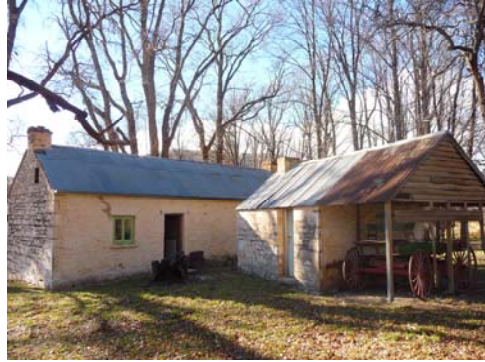
Blythburn cottage and kitchen at rear
