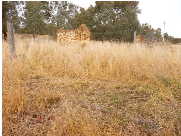
1874 homestead – extent indicated by foundations in foreground, timber beam to LHS and stone ruin to right. A stone outbuilding sits behind the homestead.
