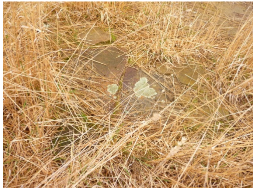
Foundation stones for what appears to be a second outbuilding near 1874 homestead
