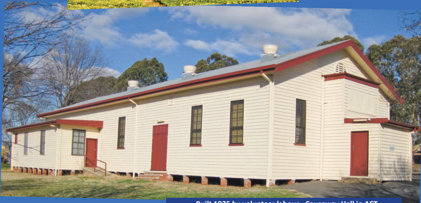
Built 1925 by volunteer labour - Causeway Hall in ACT
