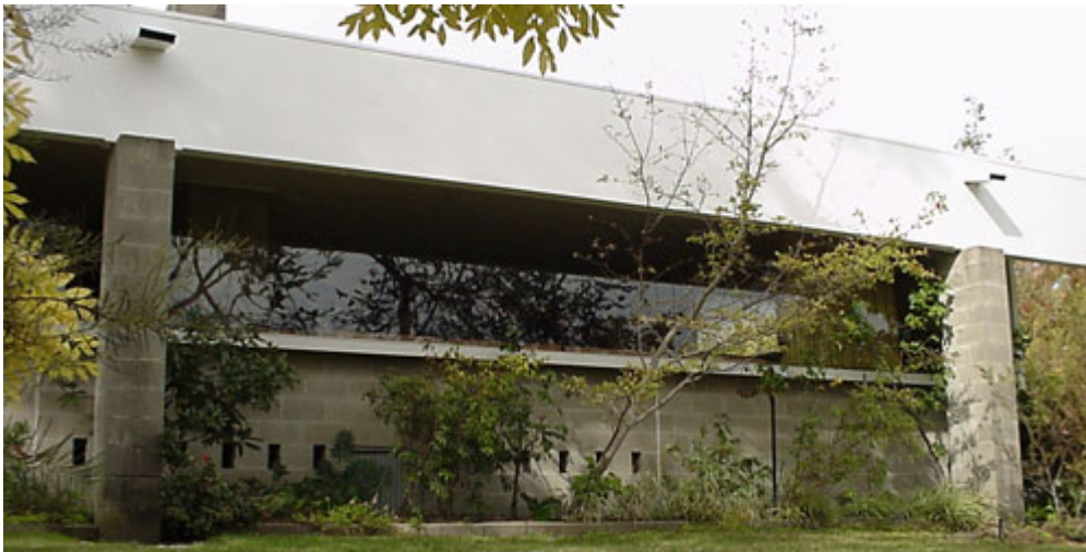
Figure 1. Front view of 1 Astley Place, Garran.
