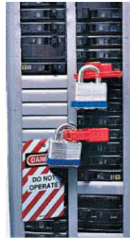
Danger tagged circuit breaker locking off devices
