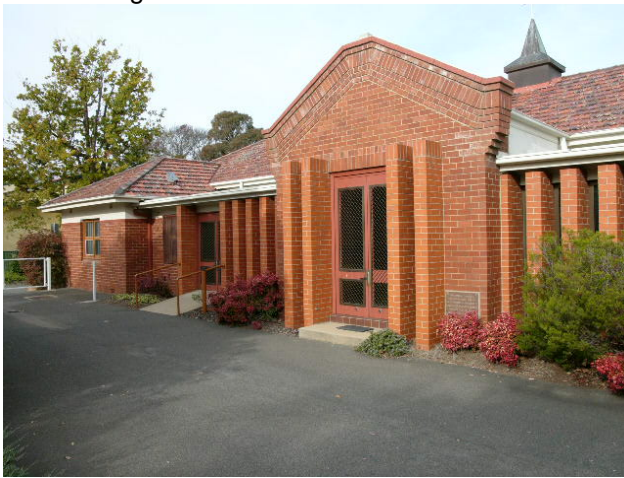
St Patrick's Church Braddon 2010 (Photograph M Cameron)
