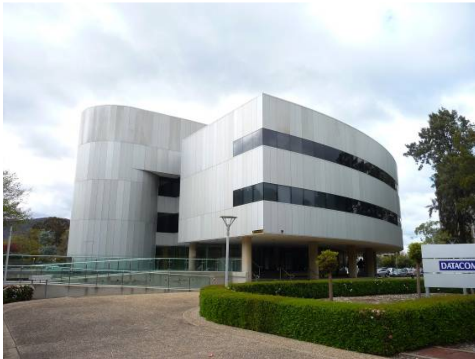
Image 3. Former Australian Automobile Association Building from Northbourne Avenue. (ACT Heritage 2013)
