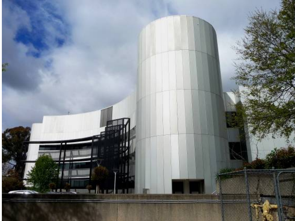
Image 4. Former Australian Automobile Association Building northern side with the black sun control scaffolding visible on the left in front of the building. (ACT Heritage 2013)
