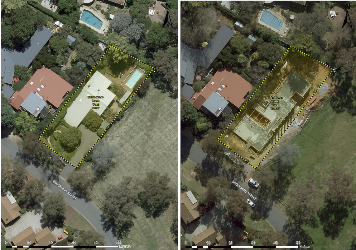
Image 1 Paral House site boundary. Left in 2021 with the original house; and right in 2022 with the new house mid-construction.
