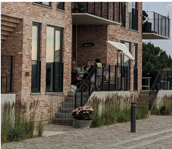
Photo 31: Slightly raised balcony with private access to street level in an urban context. Narrow planted zone softens the building edge and offers the opportunity to screen privacy further with taller planting. Design: Henning Larsen Architects
