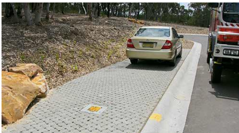
Figure 15. Hydrants and parking bays.
