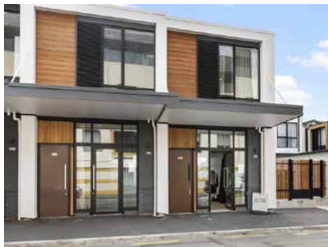
Photo 36: Generous ground floor ceiling heights allow for flexible uses such as micro-retail or a cafe.
