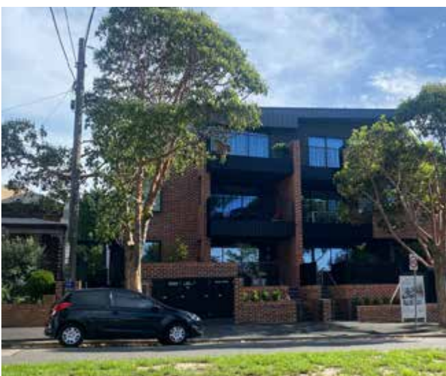
Photo 27: A stepped transition to the street provides a usable balcony for the ground floor dwellings. Hotham Hill Apartments, Melbourne VIC. Architect: MGS Architects
