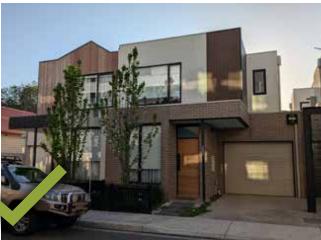
Photo 41: Setting individual garages back from the front building line reduces the visual dominance of garage doors and prioritises integrating dwellings to maintain a cohesive streetscape.
