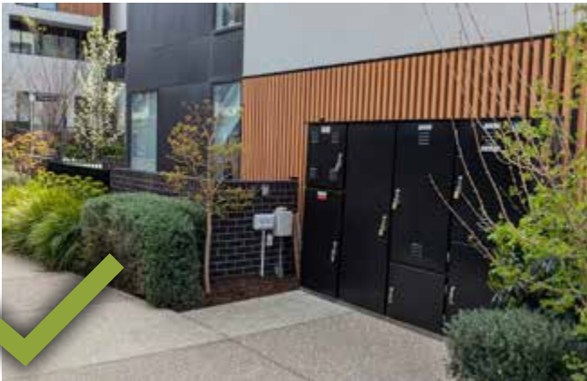
Photo 46: Co-locating infrastructure elements on the least active facade away from the street can be an efficient design outcome as this minimises negative impacts on the public realm. The Mills, Alphington, VIC. Architect: DKO Architects
