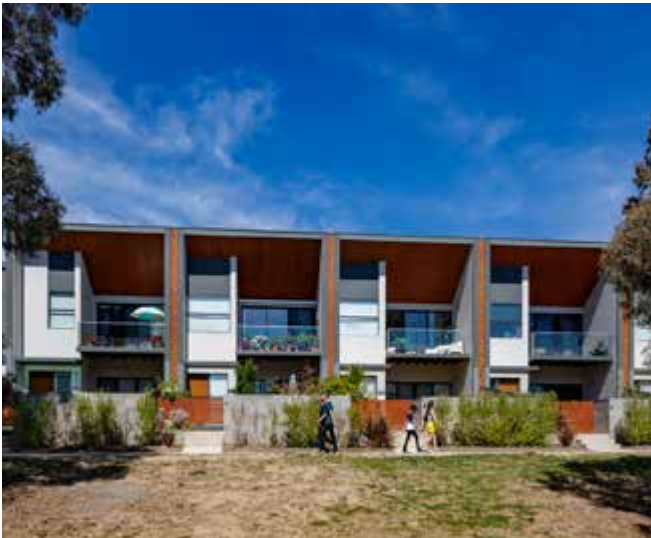
Photo 17: Terrace houses with a good quality ground floor interface can contribute to the safety and vitality of streets. Aranda Townhouses, Aranda ACT. Architect: DNA Architects.
