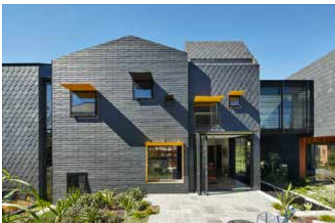
Photo 78: Architectural elements can be used to produce shade. Charles House, Melbourne VIC. Architect: Austin Maynard Architects. Photograph: Peter Bennetts
