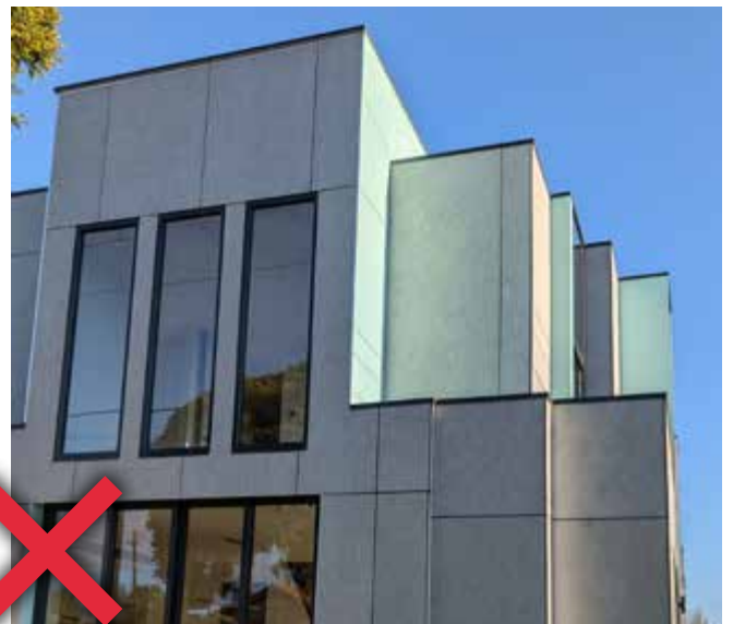
Photo 64: The excessive use of upper level setbacks and a single material makes the facade appear messy from the street.
