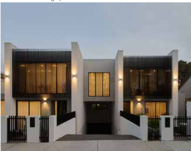
Photo 9: Parking access is sensitive to the topography and recessed from the street. Rossmoyne Townhouses, Rossmoyne, WA. Architect: C. Kairouz Architects
