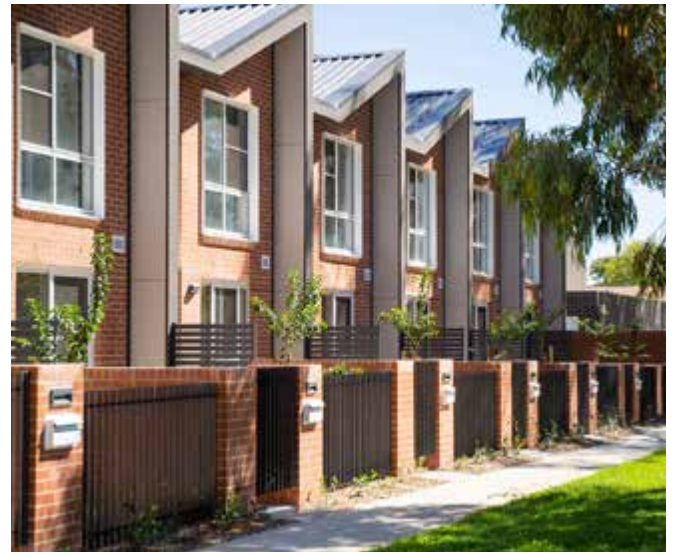
Photo 20: The use of fencing creates a clear differentiation between public and private space. The Bradfield, Downer ACT. Architect: AMC Architecture
