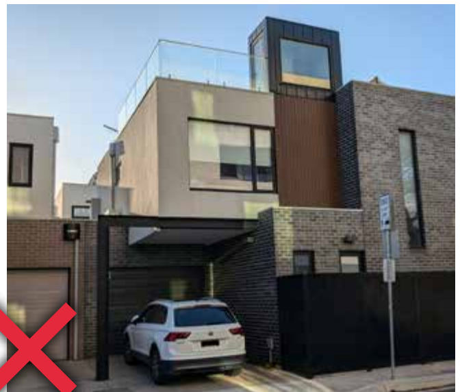
Photo 66: No windows provided in the facade which is mainly taken up by the garage door. Allowing no passive surveillance and street activation.
