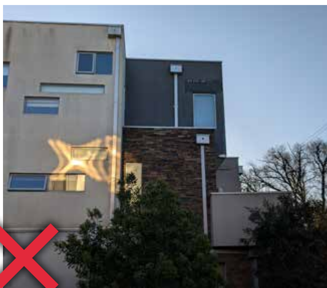
Photo 62: The excessive use of materials and a lack of clear setbacks and articulation fail to successfully define the building.
