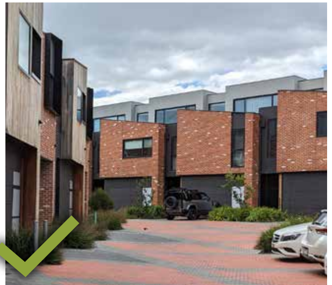
Photo 58: Articulation in roof form at the second floor. The upper level setback and modulation in form reduce the visual bulk of the third floor. Merri Green, Northcote VIC. Architect: Chamberlain Architects and Interiors
