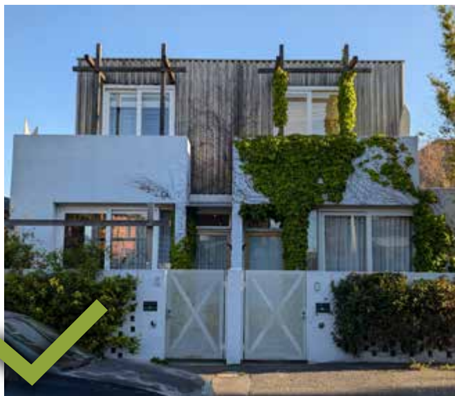
Photo 61: The contrast of timber and white brick helps to differentiate the levels of the building and is consistent with the use of setbacks and articulation. Arnold Street Townhouses, Brunswick East, VIC.
