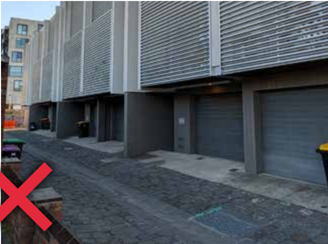
Photo 39: Garages without natural light and landscaping creates an unattractive and hostile urban environment which does not encourage other uses.
