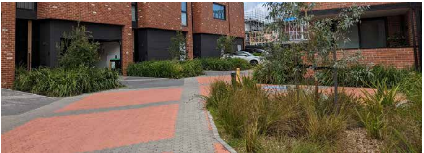
Photo 31: Permeable paving combined with green infrastructure, such as rain gardens, can help to manage runoff (reducing pollution) and reduce the risks associated with flooding and rainfall surge events.
