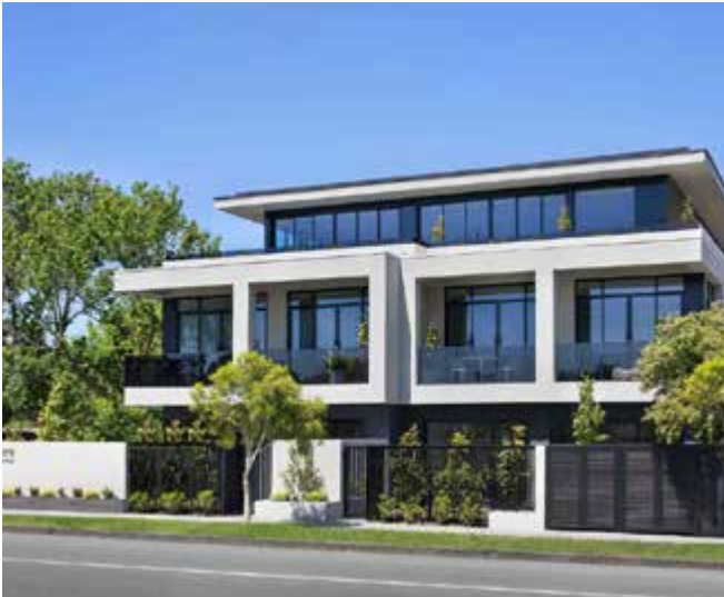
Photo 23: The use of an upper level setback minimises the visual bulk associated with the height of the building. Malvern Apartments, Melbourne VIC. Architect: C. Kairouz Architects. Photograph: Emily Bartlett
