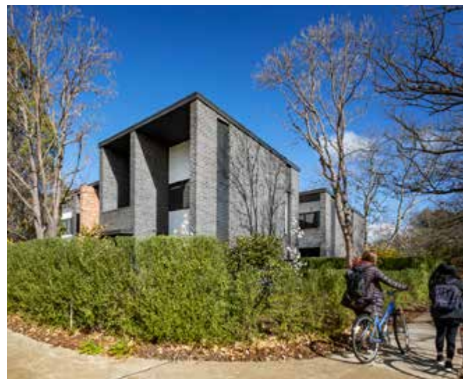
Photo 16: A simple use of articulation and materiality creates visual interest. Turner Townhouses, Turner, ACT. Architect: de Rome Architects
