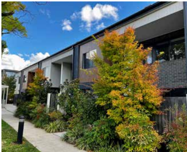
Photo 54: Planting can be highly effective at maintaining a level of privacy to dwellings facing communal areas. However, this needs to be balanced to maintain passive surveillance. Grace, Dickson ACT. Architect: DNA Architects
