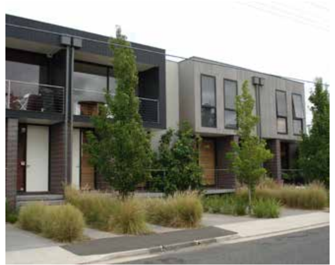
Photo 18: Architectural articulation and varied materiality can help to avoid a repetitive frontage. Townhouses, Geelong, VIC.
