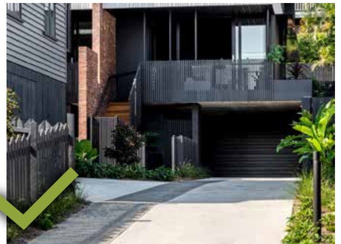
Photo 42: A shared garage has been integrated into the secondary facade of one dwelling to reduce driveway crossovers and hard stand to allow for additional landscaping to soften edges. Longfellow Terraces, Norman Park QLD. Architect: Refresh Studio for Architecture. Photograph: Catherine Schusler
