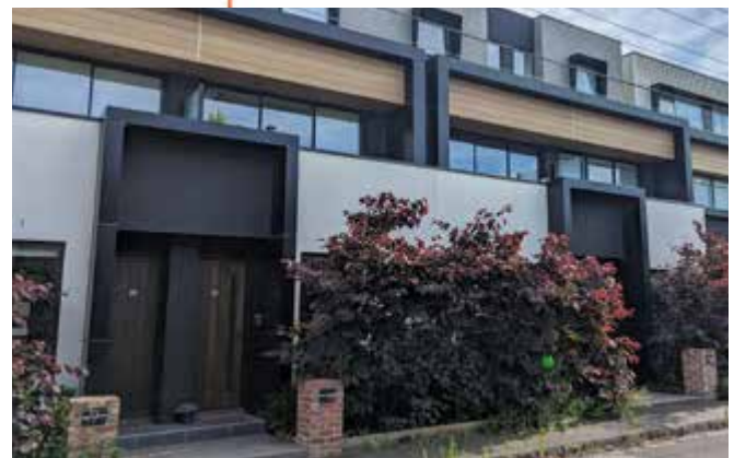
Photo 69: Narrow front setback with planted area in front of glazed windows and high window sills to mitigate privacy risk on ground floor level.
