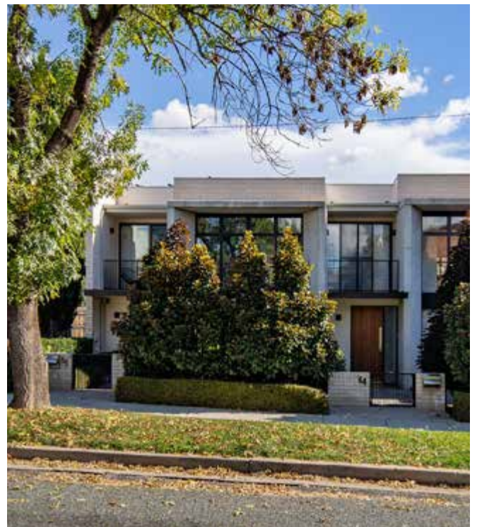
Photo 33: Slightly raised front-facing courtyards to ground-floor townhouses units provides activation of the street while maintaining privacy and passive surveillance. Design: Stewart Architecture.
