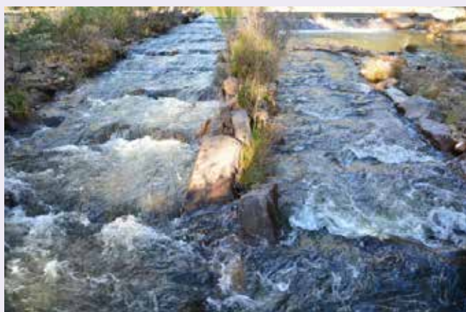
Fishway at Vanitys Crossing, Cotter River (M. Jekabsons)
