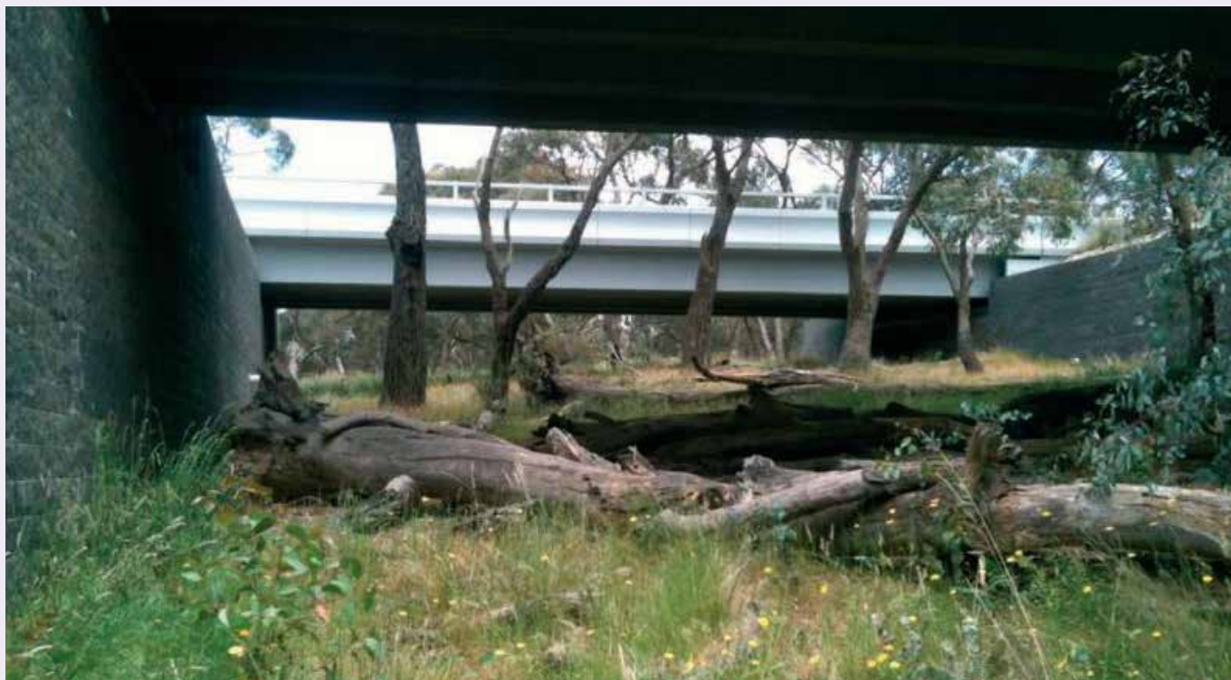
Fauna underpass on the Calder Freeway. Source: VicRoads Fauna sensitive road design guidelines.
